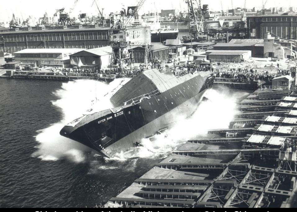
Side launching of the hull of fish trawler at Gdynia Shipyard
